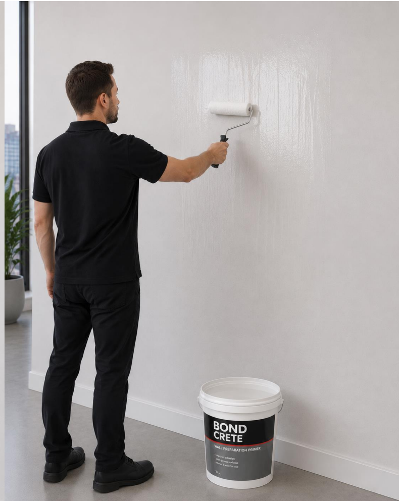
Step 2 Prime the wall with BondCrete or similar if required
