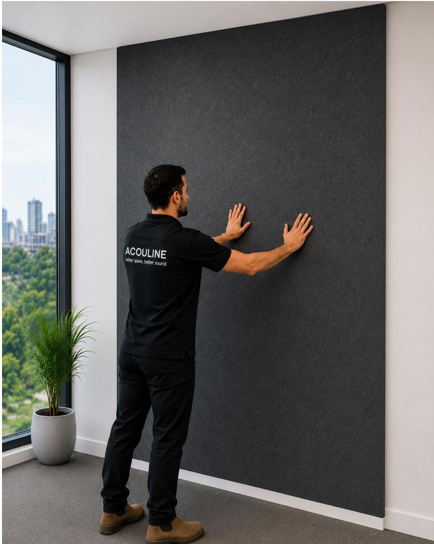
Step 7 Carefully position the panel and press firmly across the entire surface using even pressure.
