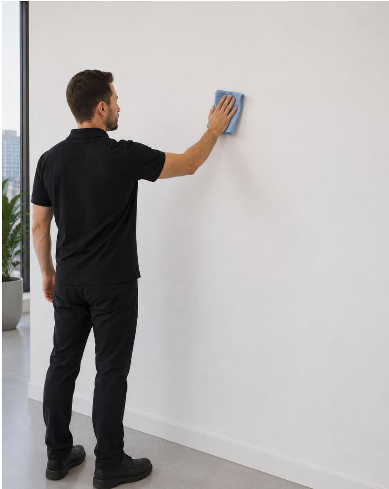
Step 1 Clean the wall thoroughly with a clean cloth and warm soapy water
